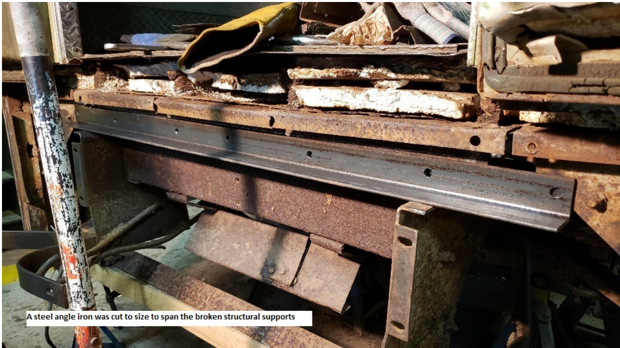
A steel angle iron was cut to size to span the broken structural supports
